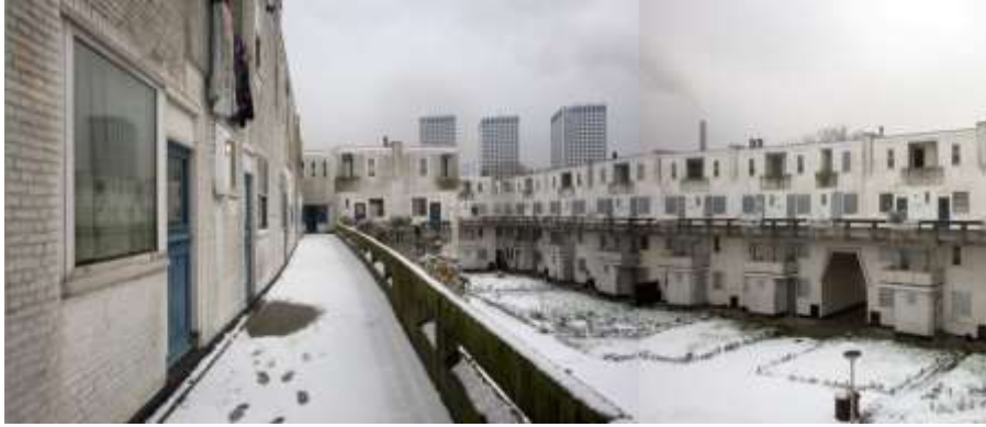
Figure 4: The Justus van Effen Residential Complex 2010 before Intervention
